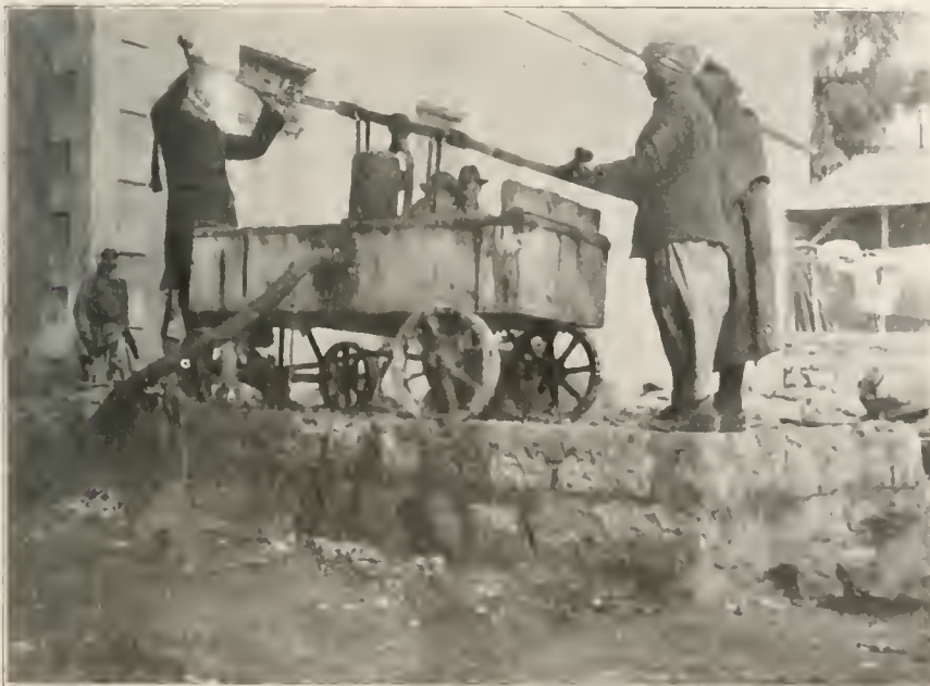
Pumping the sewage from a hospital cess pit to the tank in which it is carted away.
